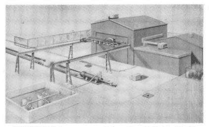
ARTIST'S SKETCH shows arrangement of new Dynamic Stock Test Facility planned for Sandia Laboratory's Area III. In the center, underneath the bridge crane, is a sled being propelled down the 180-ft. track.
